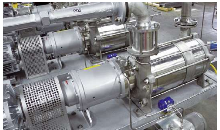
VHCM (ChemTAL) liquid ring vacuum pump as per TA Luft with a pump monitoring system used for solvent recovery.
